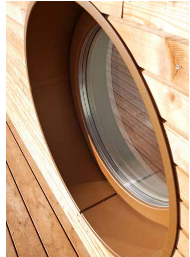
Kindergarten in Moosdorf
